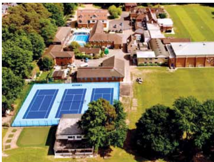
New Tennis Courts, installed in 2020
